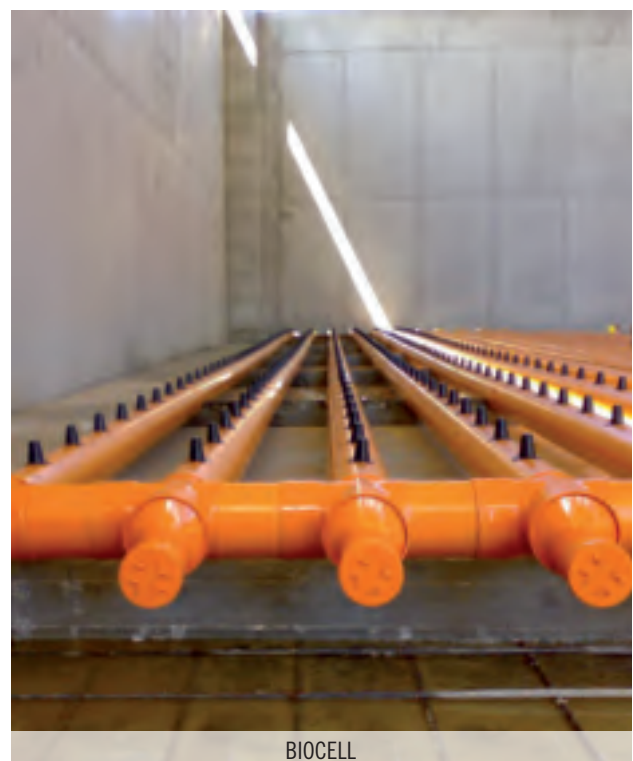
BIOSTABILIZATION AIR PRETREATMENT PLANT
